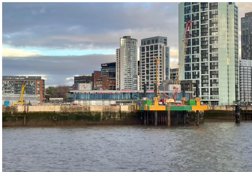
The new Liverpool Ferry Terminal under construction, but £52 million over budget.
